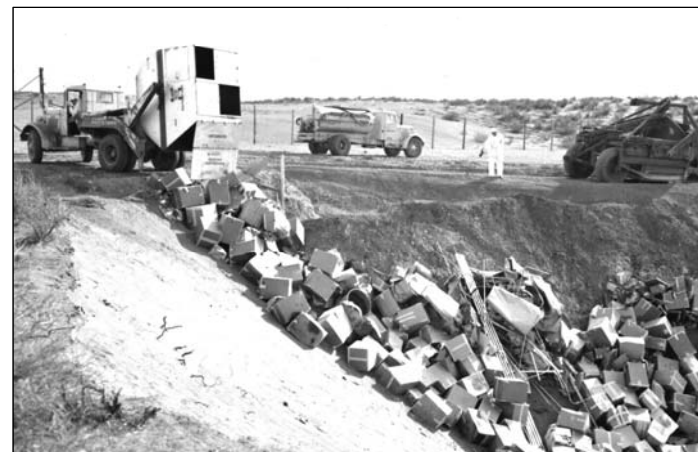
Waste was dumped directly into trenches at the 618-10 Burial Ground.
