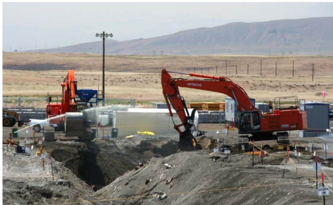
Trench excavation began in April 2011.
