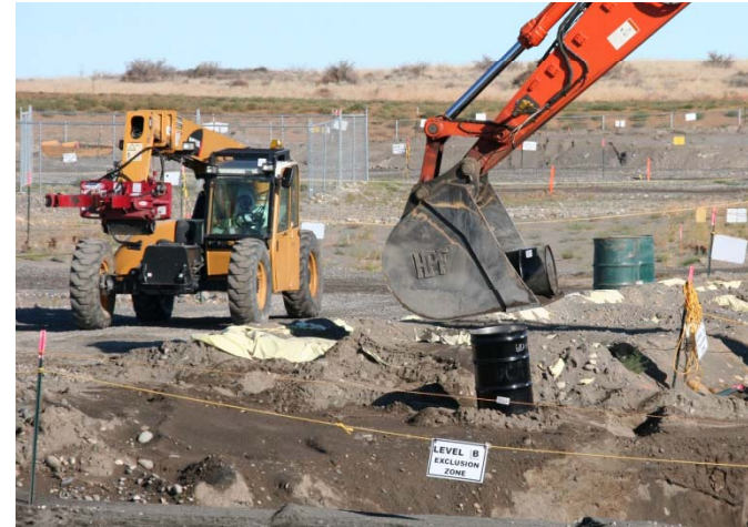
Mock-up exercises were conducted before the start of trench remediation.
