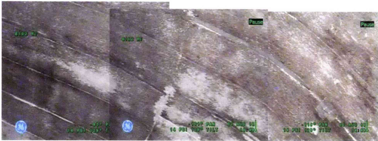
Figure 8-2: Compilation of Photographs of Tank 241-B-102 Dome
