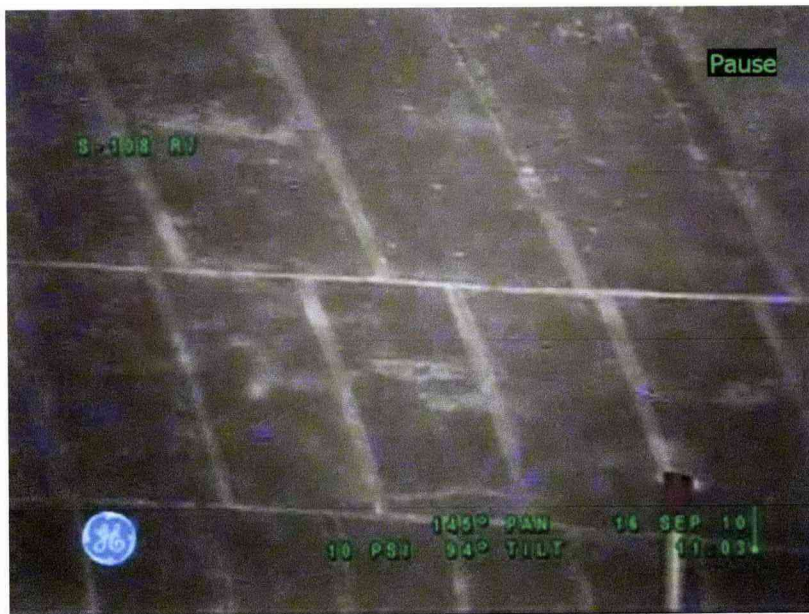
Figure 14-1: Tank 241-S-108 Concrete Dome
