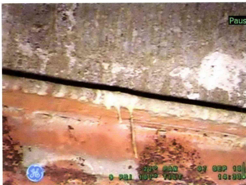
Figure 10-3: Tank 241-C-110 Steel Liner
