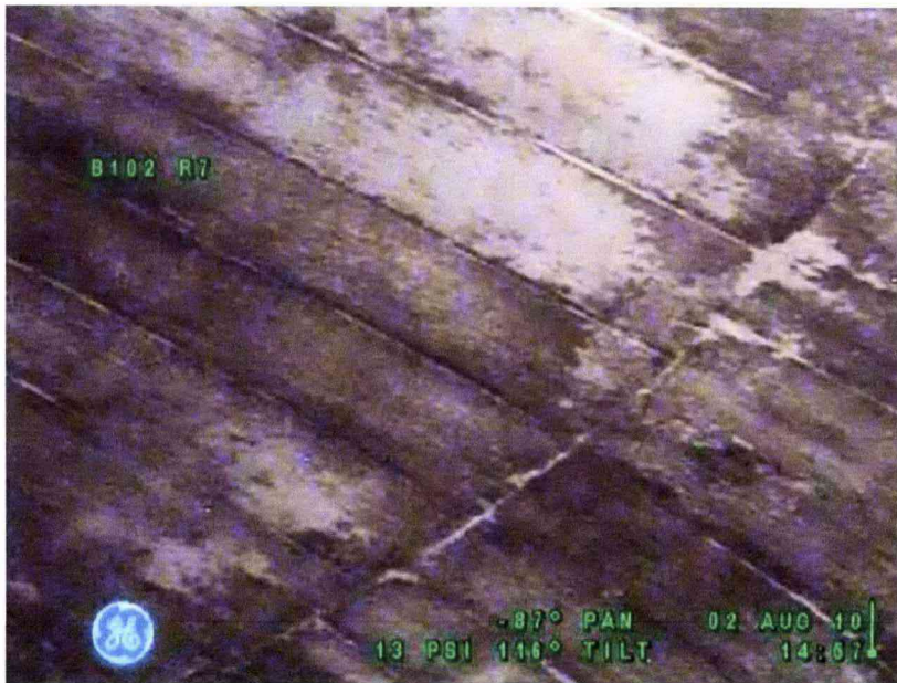
Figure 8-1: Tank 241-B-102 Concrete Dome
