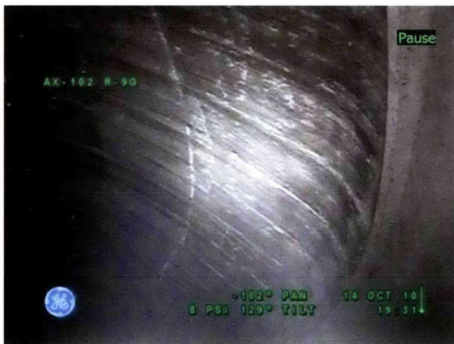
Figure 7-1: Tank 241-AX-102 Concrete Dome
