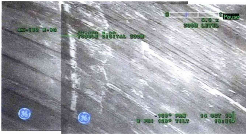
Figure 7-2: Compilation of Photographs of Tank 241-AX-102 Dome
