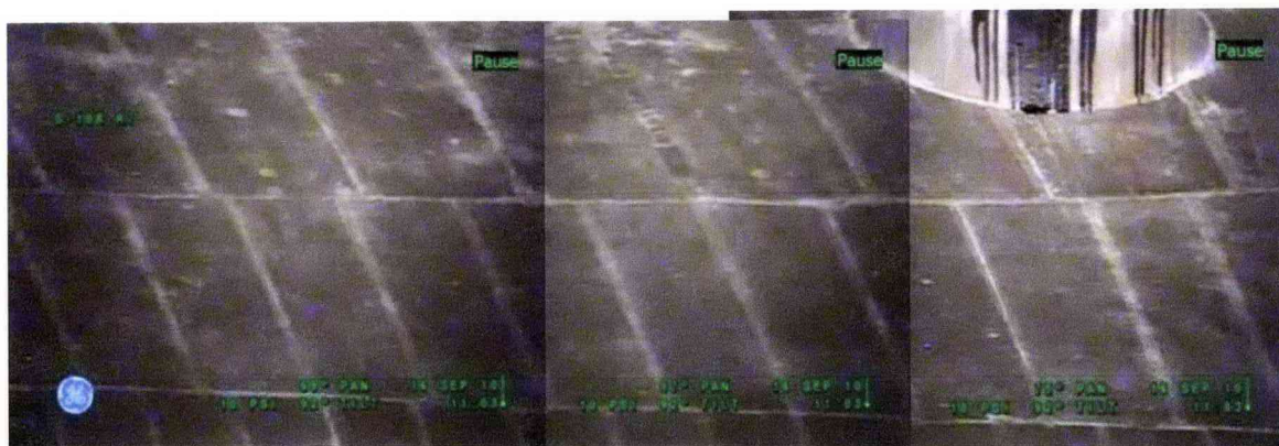
Figure 14-2: Compilation of Photographs of Tank 241-S-108 Dome
