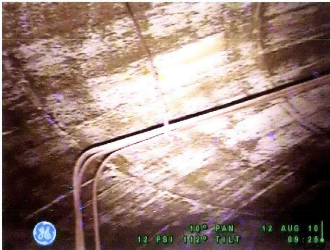
Figure 6-1: Tank 241-A-106 Concrete Dome
