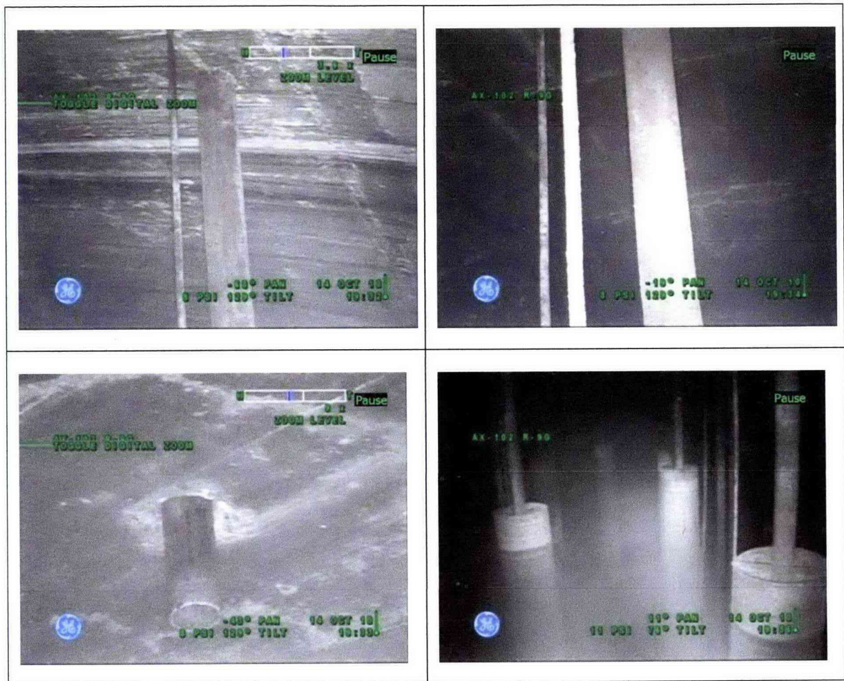
Figure 7-5: Tank 241-AX-102 In-Tank Equipment/Risers
