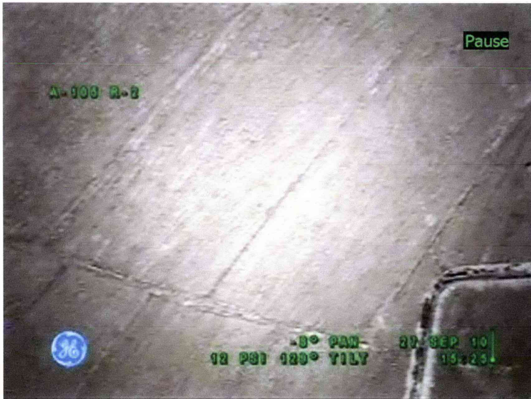
Figure 5-1: Tank 241-A-105 Concrete Dome
