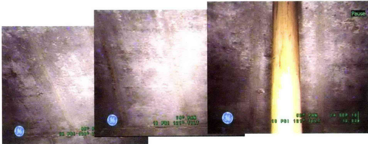
Figure 12-2: Compilation of Photographs of Tank 241-S-103Dome
