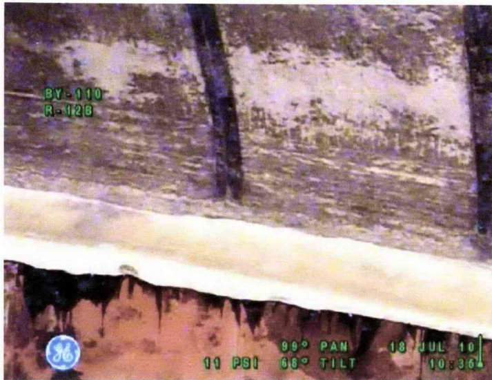
Figure 9-5: Tank 241-BY-110 Steel Liner
