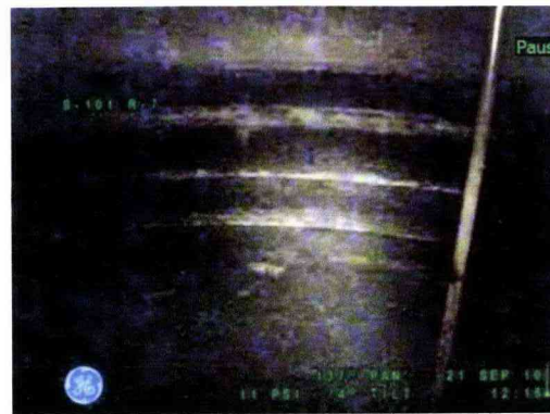
Figure 11-5: Tank 241-S-101 Steel Liner
