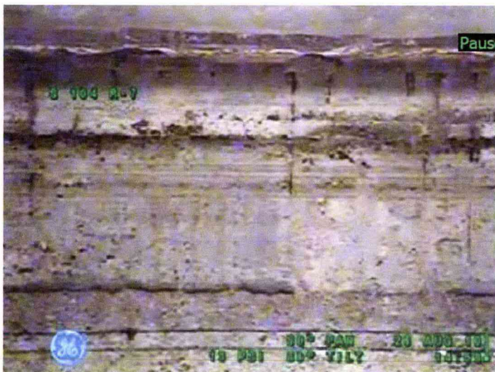
Figure 13-3: Tank 241-S-104 Steel Liner
