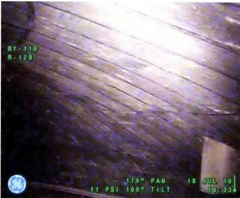
Figure 9-1: Tank 241-BY-110 Concrete Dome
