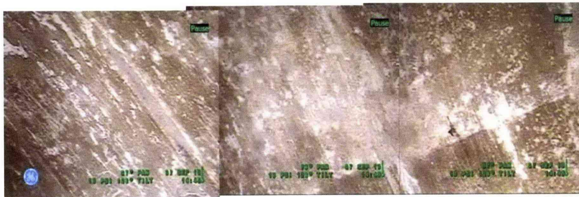
Figure 10-2: Compilation of Photographs of Tank 241-C-110 Dome
