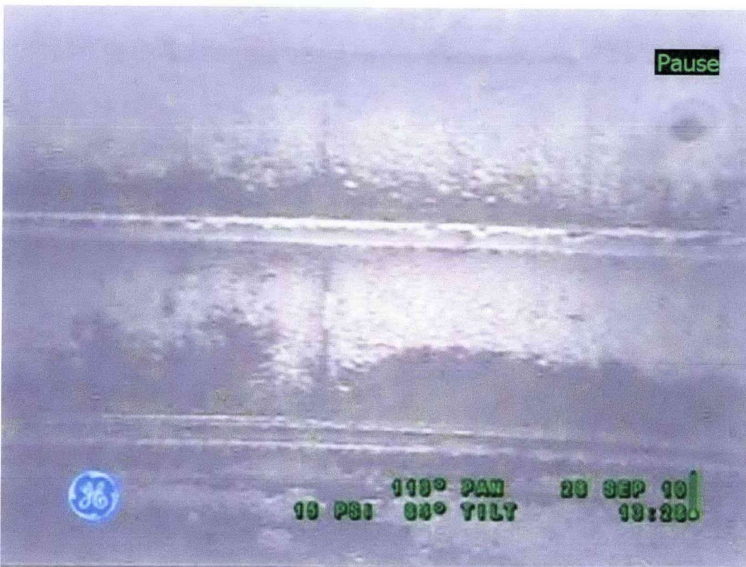
Figure 5-4: Tank 241-A-105 Steel Liner
