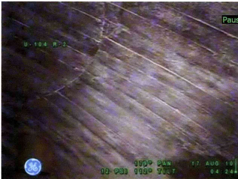
Figure 16-1: Tank 241-U-104 Concrete Dome
