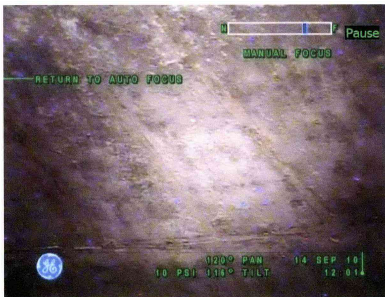
Figure 12-1: Tank 241-S-103 Concrete Dome
