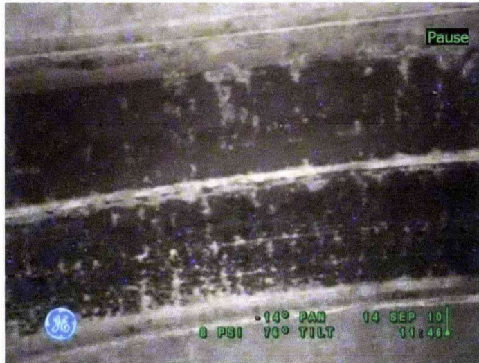
Figure 12-5: Tank 241-S-103 Steel Liner
