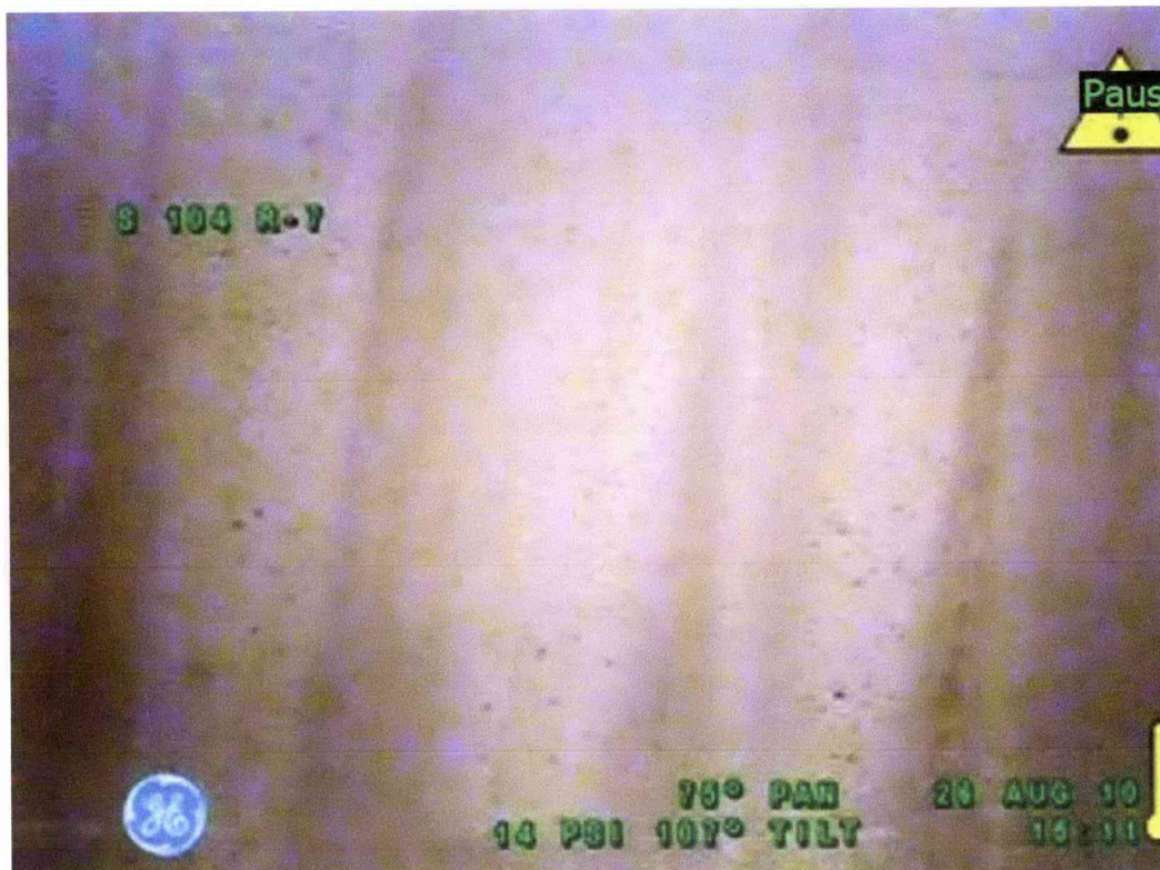
Figure 13-1: Tank 241-S-104 Concrete Dome
