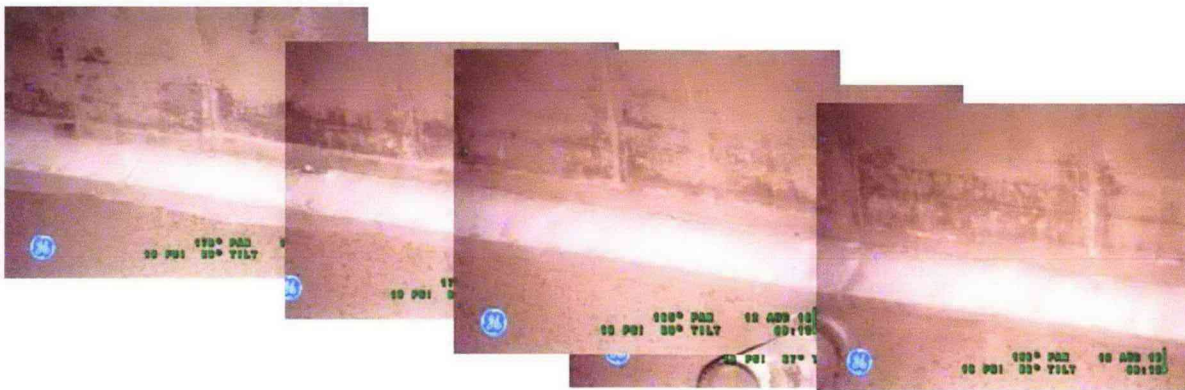
Figure 6-4: Compilation of Photographs of Steel Liner Tank 241-A-106
