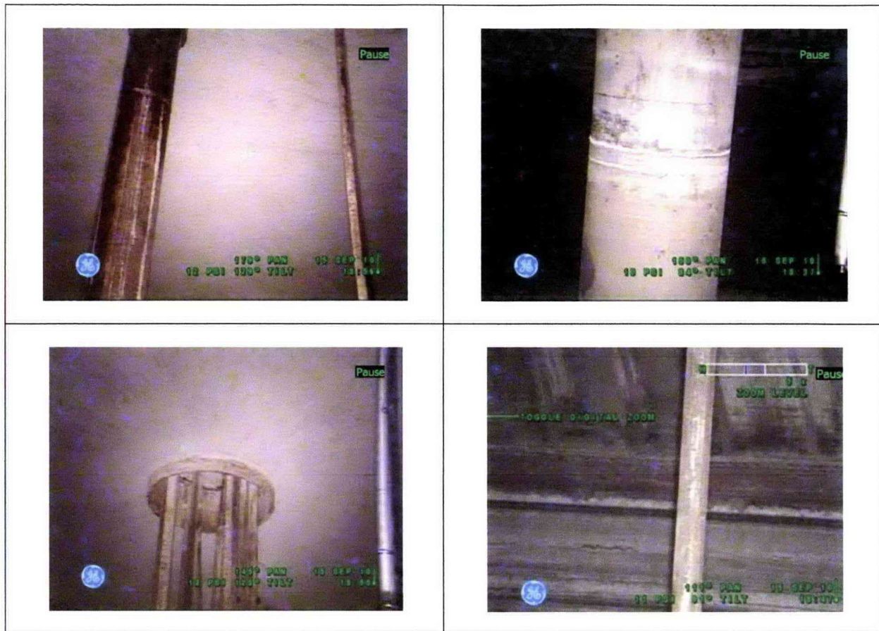
Figure 15-6: Tank 241-SX-101 In-Tank Equipment/Risers
