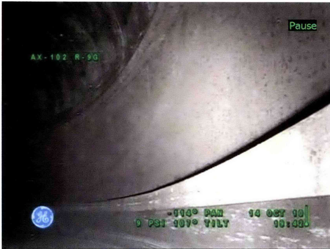
Figure 7-4: Tank 241-AX-102 Steel Liner
