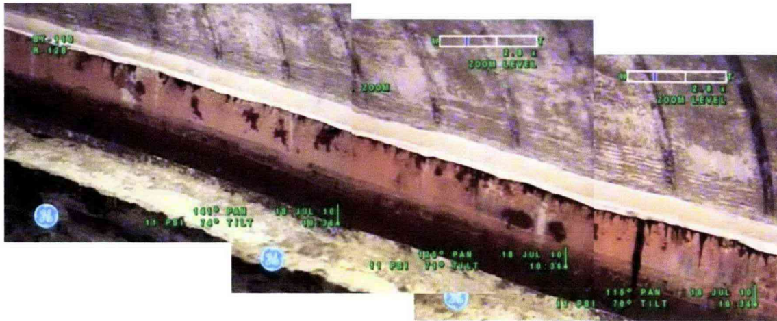
Figure 9-6: Compilation of Photographs of Steel Liner Tank 241-BY-110
