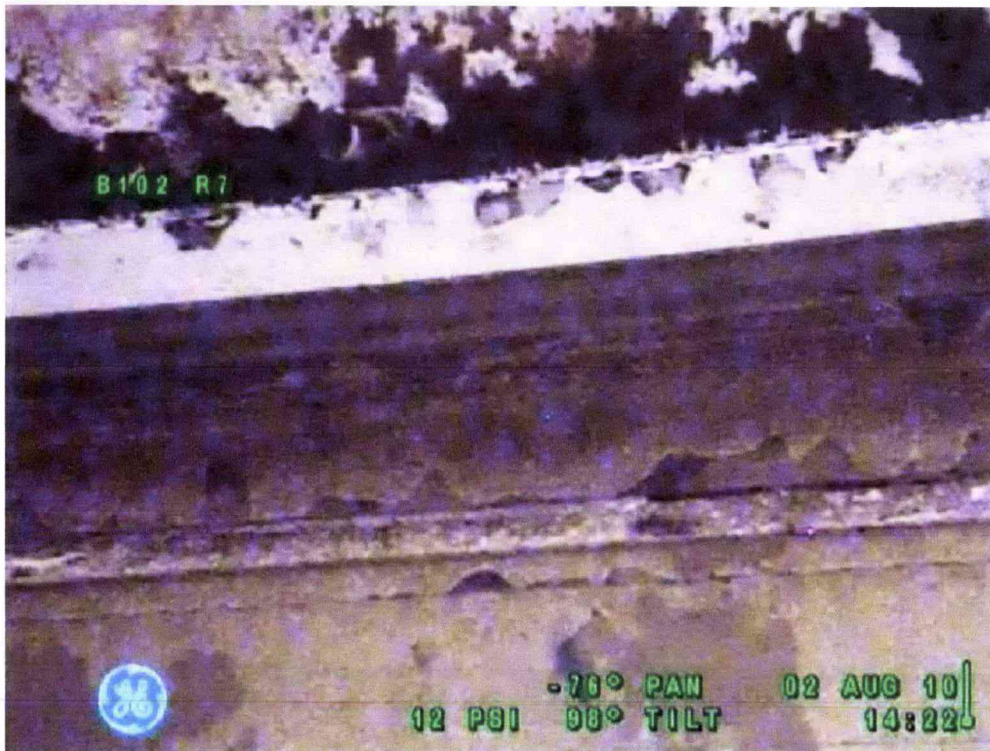
Figure 8-3: Tank 241-B-102 Steel Liner
