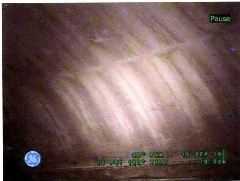
Figure 15-1: Tank 241-SX-101 Concrete Dome
