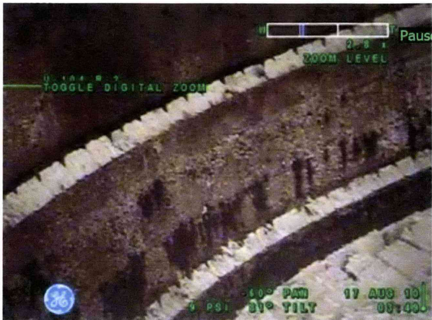
Figure 16-5: Tank 241-U-104 Steel Liner
