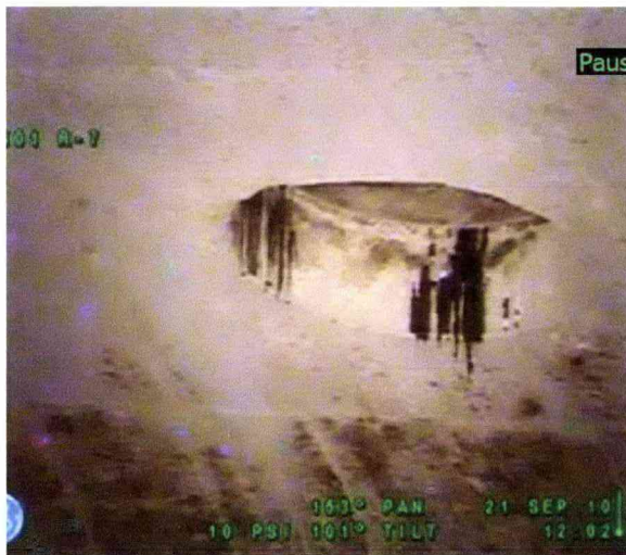
Figure 11-1: Tank 241-S-101 Concrete Dome
