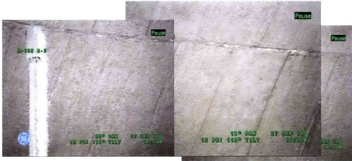
Figure 5-2: Compilation of Photographs of Tank 241-A-105 Dome
