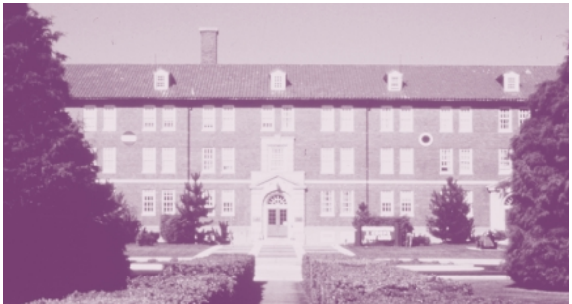
HEADQUARTER I CORPS IS ONLY ONE OF THE MANY BUILDINGS AT FORT LEWIS IN TACOMA, WASHINGTON, THAT WAS MADE MORE ENERGY-EFFICIENT THROUGH FEMP AND SEP SPECIAL PROJECTS.
