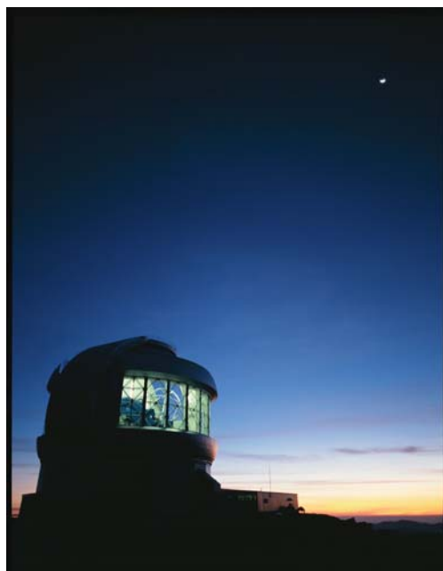
The Gemini South telescope on Cerro Pachon in Chile prepares for the beginning of observation. The telescope is visible through the three-story-high vents on the rotating dome, which allow a strong air flow across the telescope to provide good image quality. Credit: Gemini Observatory/Association of Universities for Research in Astronomy.
