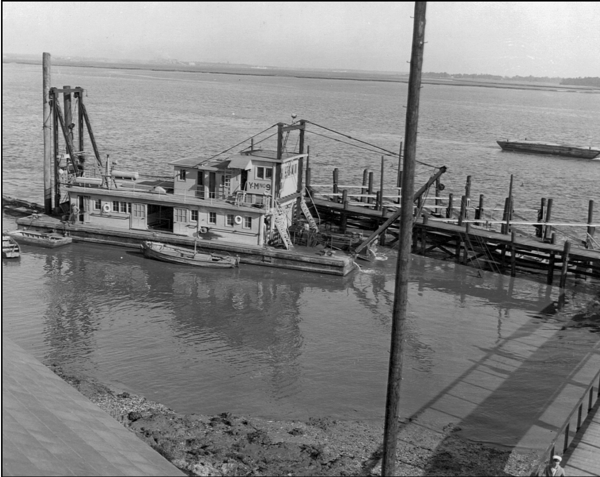
Figure 37. Cutterhead-type dredge, YM-09, 1943 (Bureau of Aeronautics 1943).
