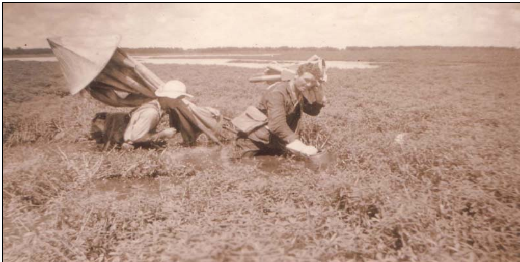
Figure 4.2. Pete Rogers and Another Crew Member Walking through the Swamp to Set Up Torsion Balance Equipment for Seismic Exploration. Photo Courtesy of Pete Rogers, OOGHP.
