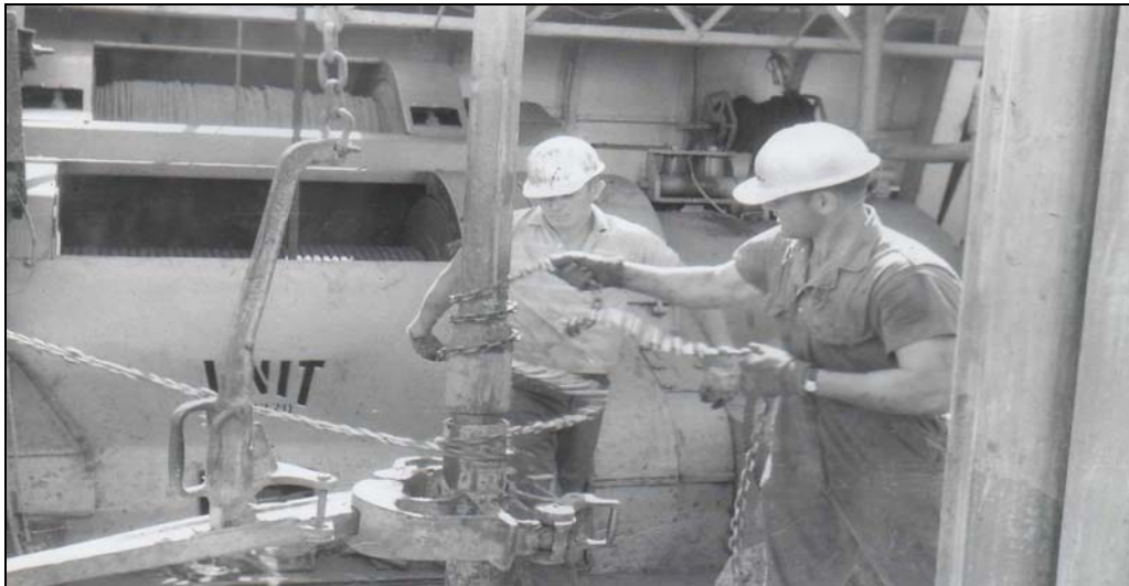
Figure 6.1. Kenneth Viator (right) and Jerry Salters Throwing the Chain on a Drilling Rig. Photo Courtesy of Kenneth Viator, OOGHP.
