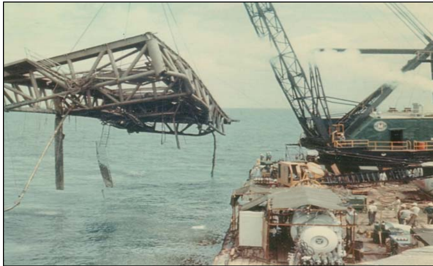
Figure 6.8. Salvaging a Platform after a Hurricane, 1966. Photo Courtesy of Jim Burgess, OOGHP.
