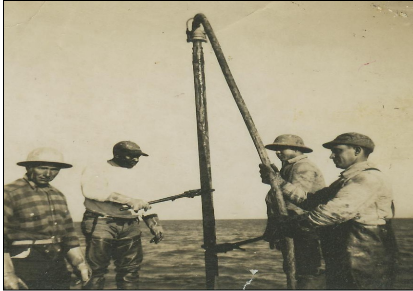
Figure 5.13. Seismic Crew Drilling Holes for Dynamite. Photo Courtesy of Nelson Constant, OOGHP.
