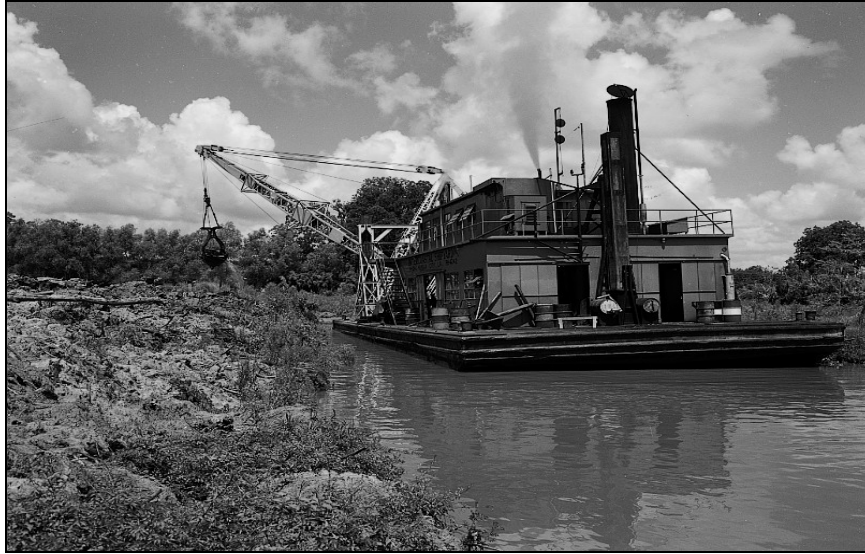
Figure 6.11. Intercoastal Shipyard Dredge Barge Digging Canal, 1956. Photo Courtesy of Jesse Grice Collection, Morgan City Archives.
