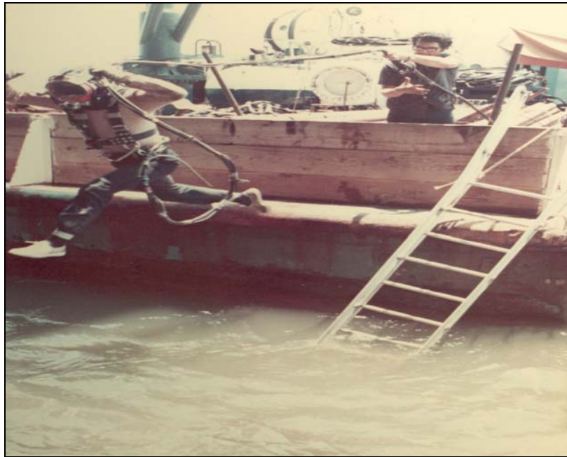
Figure 6.6. Diver Entering the Water While His Tender Stands on Deck Managing His Air Hose. Photo Courtesy of Lynda Miller, OOGHP.
