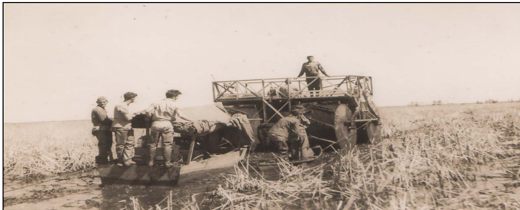
Figure 5.5. Using a Marsh Buggy to Haul People and Supplies through the Marsh. Photo Courtesy of Russell Poencot, OOGHP.
