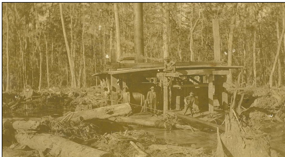
Figure 2.3. Logging in the Swamps around Morgan City. Photo Courtesy of Bernie Overhultz, Morgan City Archives.
