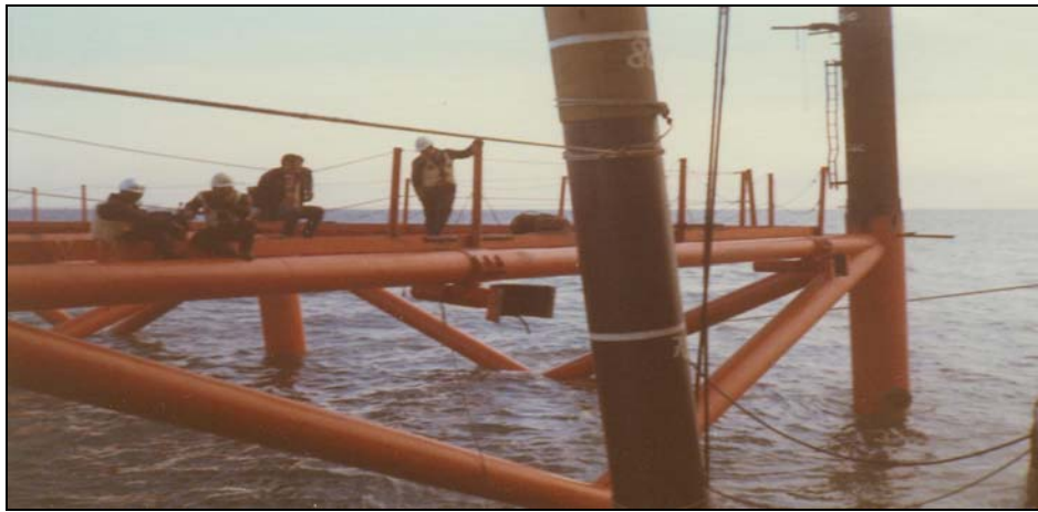
Figure 6.3. Preparing to Remove a Jacket Leg from a Platform Skeleton. Photo Courtesy of Joseph Schouest, OOGHP.
