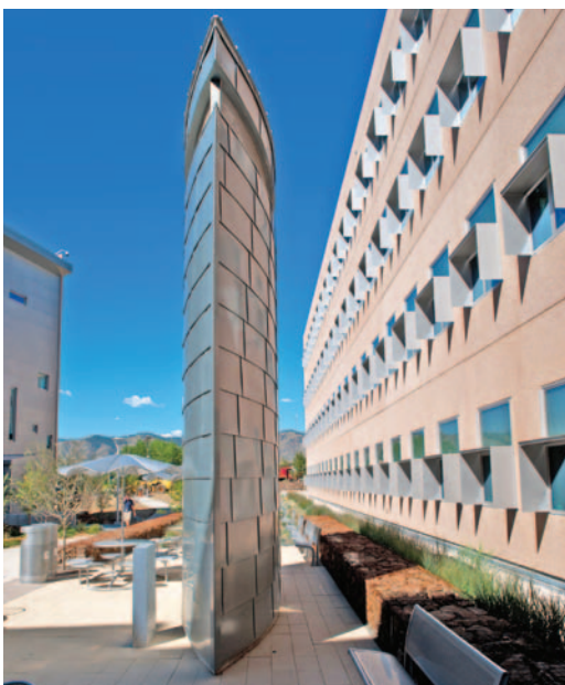
Figure 21. Data center air intake. Photo by Dennis Schroeder, NREL/PIX 19220
