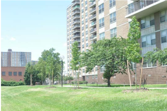
Spring Creek Towers where $6 million in ARRA funds is retrofitting over 5,000 apartments. Photo: CEC
