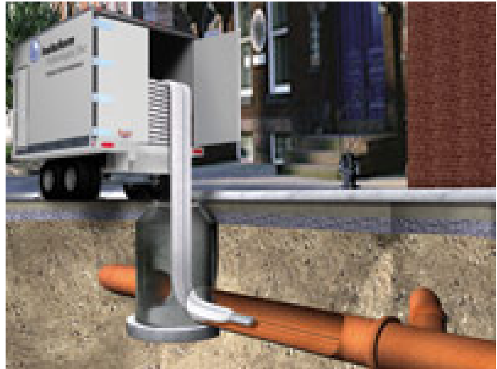
Insertion of an Inverted Liner
