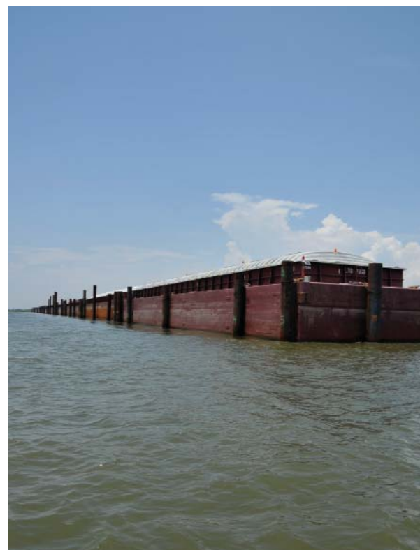
RIGOLETS CHANNEL, La. – Barges are affixed together in a long line to act as a massive boom in an effort to keep tar balls from making their way into Lake Pontchartrain. Photo courtesy of U.S. Coast Guard
