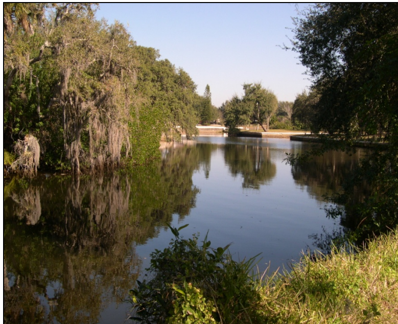
Figure 5.13. Development in the watershed; perennial stream; low levees; well-packed bed material; minor obstructions from concrete, riprap, roots; sandy clay banks; moderately steep banks; heavily vegetated or protected banks; no mass wasting; moderately well aligned (downstream from bend). R = 57 = Good (FHWA 2006).
