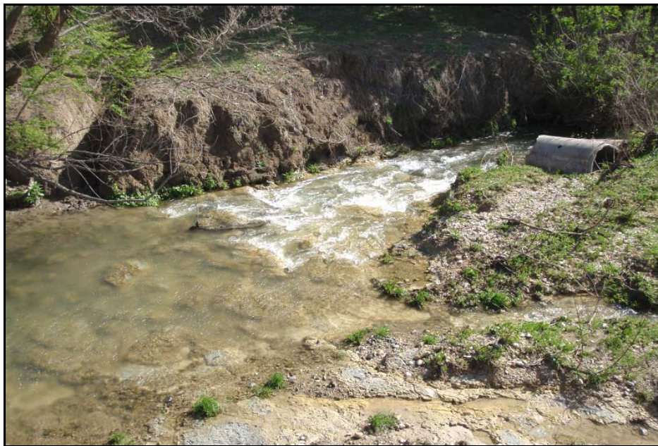
Figure 2.13. Stream channel with erodible rock bed and semi-cohesive banks.
