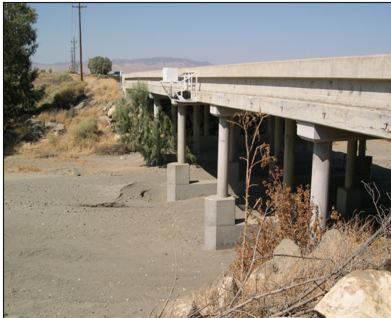
Figure 5.12. Cattle and farming activity; flashy flows; braiding; small loose bed material; minor obstructions; noncohesive bank material; some woody vegetation; limited mass wasting downstream from channel bend; meander bend 66 ft (20 m) upstream. R = 110 = \text{Fair} (FHWA 2006).
