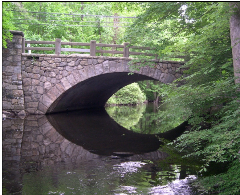
Figure 5.14. Stable watershed; perennial stream; mild meanders; no entrenchment; large, packed bed material; no obstructions; cohesive bank material; heavily vegetated banks with vertically oriented trees; little bank cutting; no mass wasting; well aligned with bridge. R = 44 = Excellent (FHWA 2006).
