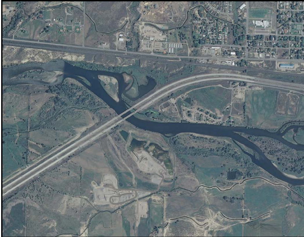
Figure 5.21. Aerial image of Interstate 70 over the Colorado River.
