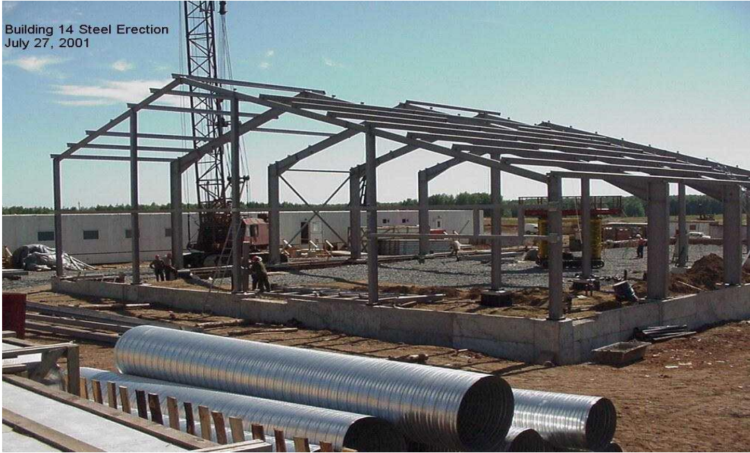
Figure C-2. Warehouse (Building 14) during construction
