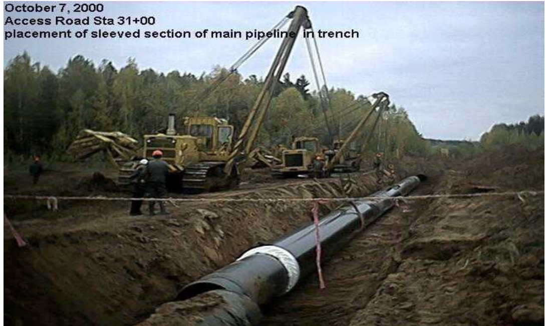
Figure C-5. Placement of natural gas pipeline
