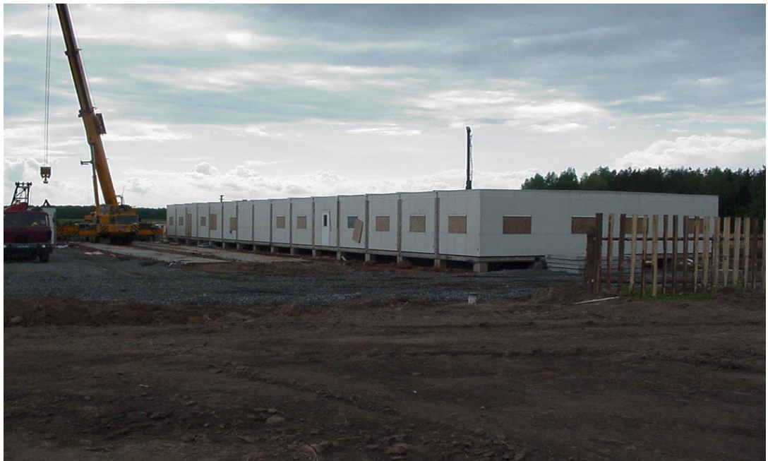
Figure C-1. Administrative building (Building 5) during construction
