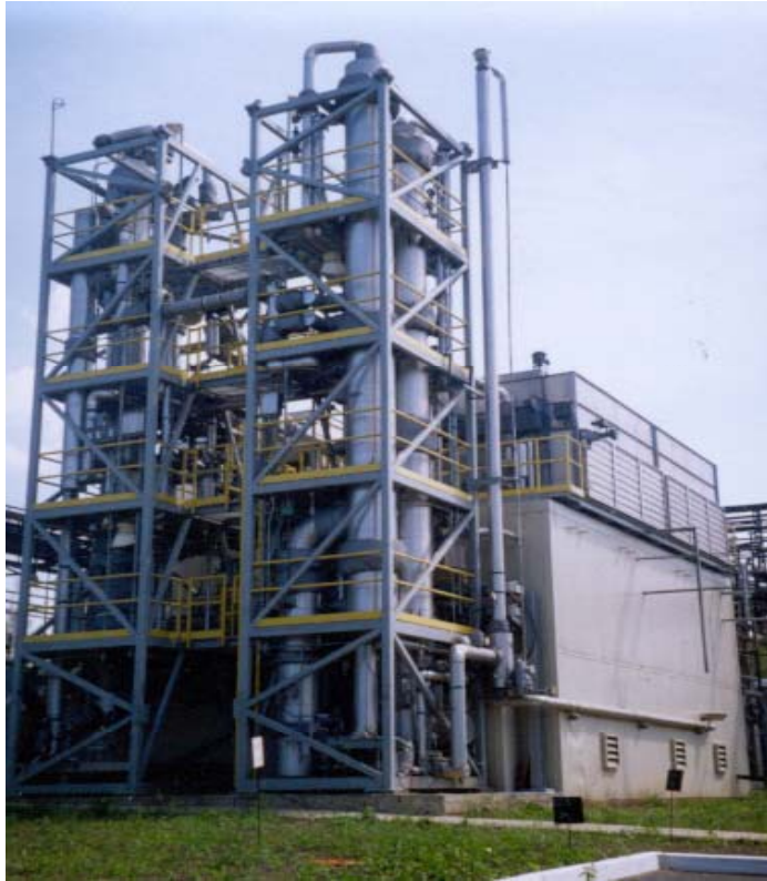
Figure D-3. Exterior of One of the Two Heptyl Disposition Units
