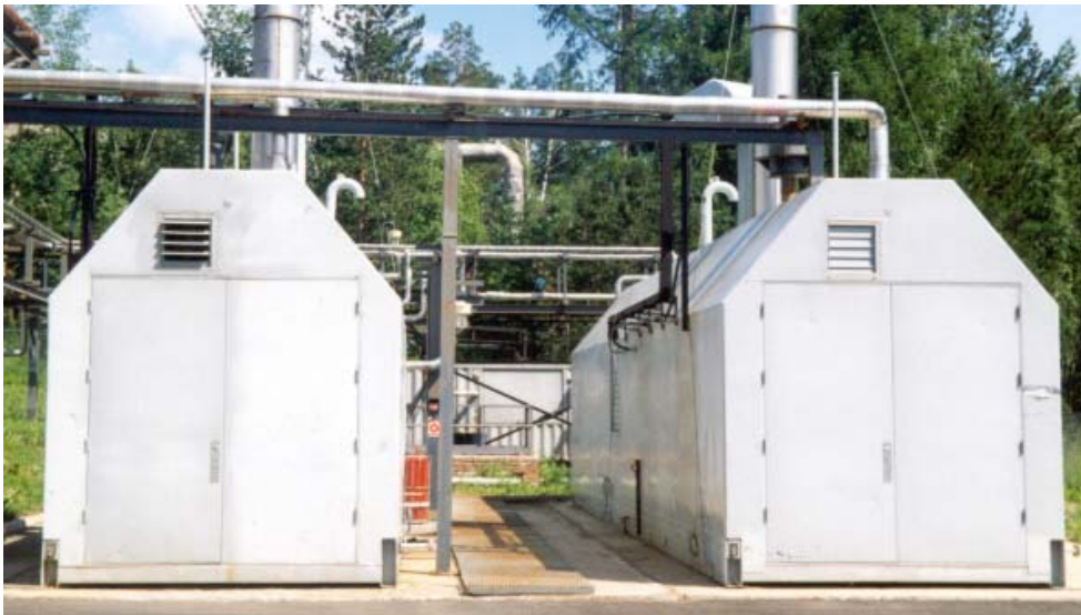
Figure D-6. Steam Generator Rooms (One for Each Disposition Unit)
