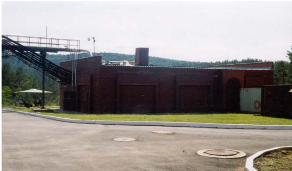
Figure D-7. Exterior of the Computer Process Control and Water Treatment System Building
