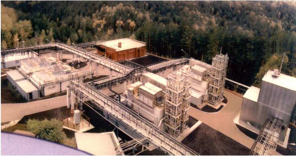
Figure D-1. Aerial view of the Heptyl Disposition Systems and Infrastructure
