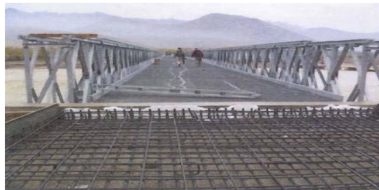
Figure 3. Nearly-Complete One-Lane Regak Bridge
