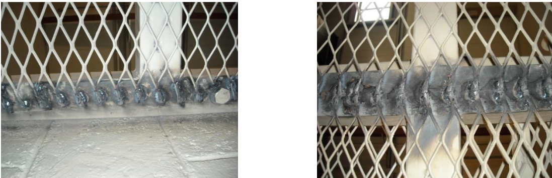
Figure 3. Re-Welded Cell Doors
