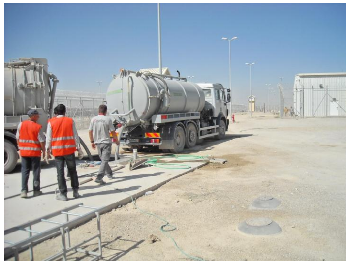
Figure 6. Trucks Collect Sewage
