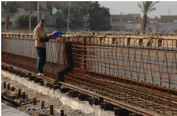
Figure 6: Bridge construction project in Iraq.
