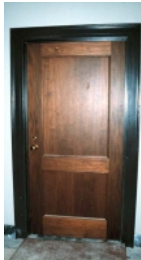
Fig. 22: 90 minute kalamein door closely matches original paneled stair doors at the Federal Trade Commission building, Washington, DC.
