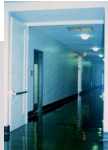
Fig. 12: Cross-corridor doors at the Federal Trade Commission building in Washington, DC, span all but 28 inches of the 10 foot wide corridor and 1 foot of the floor to ceiling height. (National Capital Region)
