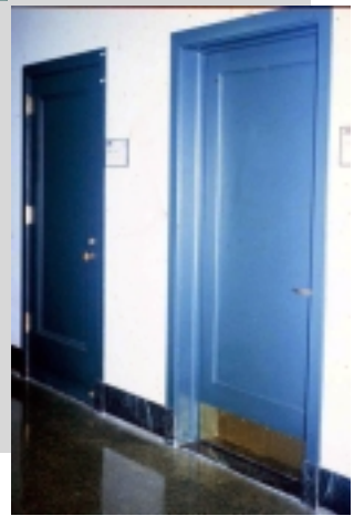
Fig. 21: Ariel Rios Building, Washington, DC. 90 minute true paneled wood door matching original corridor doors.
