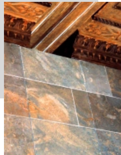
Fig. 17: Detail of faux marble painted door cover and ceiling tracks painted to match glazed bronze finish of coffers.
