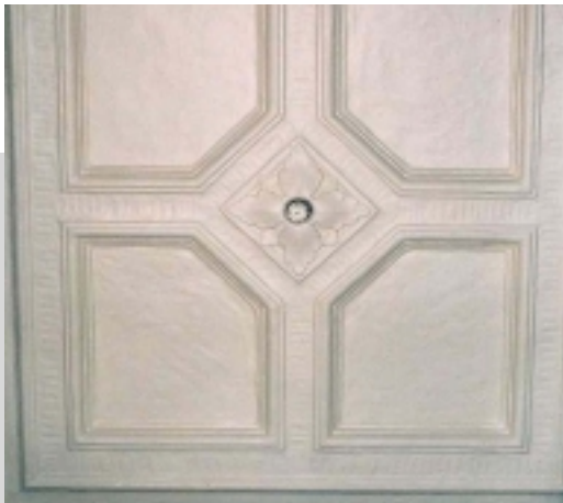
Fig. 10: Glass bulb sprinkler head mimics ceiling rosettes in the GSA Central Office building Administrator's Suite. Washington, DC.
