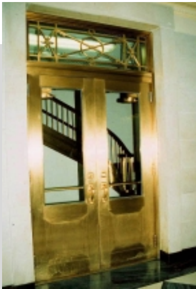
Fig. 20: Bronze and glass stair doors at the Dept. of the Interior building will be retrofitted with Superlite XL rated glass.
