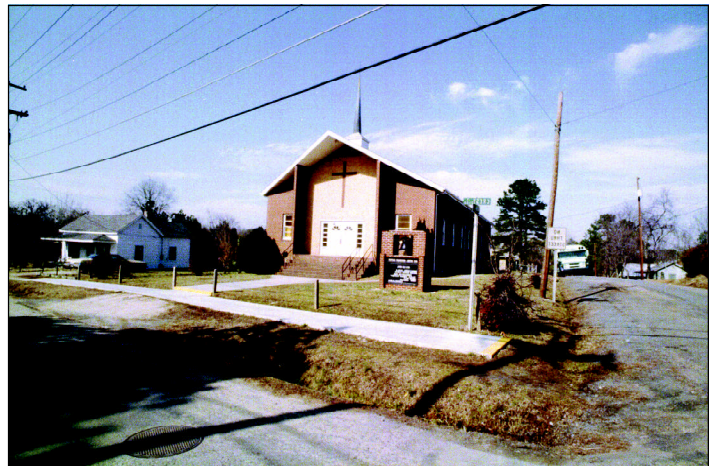
The New Bethel Baptist Church, built in 1965, was the focus of community life in Crest Street, Durham, NC. The church is shown as it was before the project.
