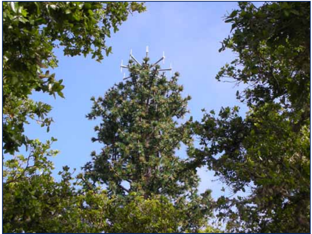
Rescue 21's first monopine tower was designed to blend in with the scenic surroundings at Big Sur's Post Ranch Inn. Photo courtesy of Lee Wilmany with General Dynamics Information Technology.
