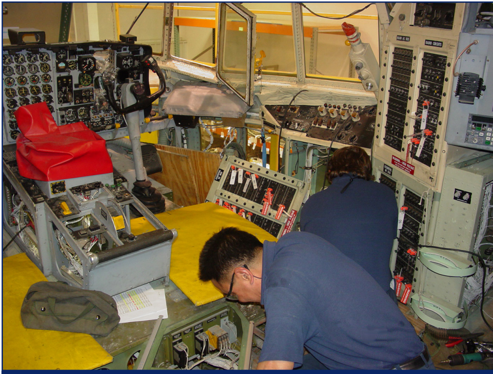
Shown here is the installation of DF-430 on board an HC-130H during overhaul at the HC-130H heavy maintenance facility in Elizabeth City, N.C. U.S. Coast Guard photo by Cmdr. Randy Hartnett
