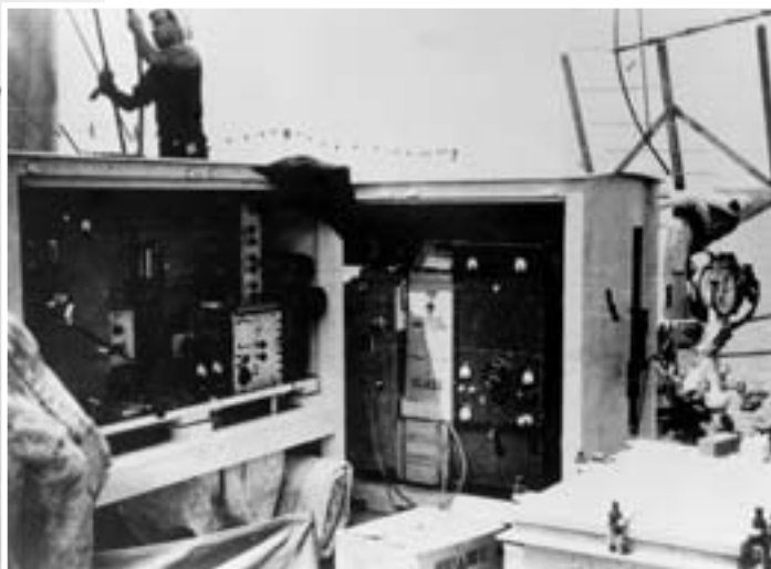
Testing radar on board USS Leary, 1937.
