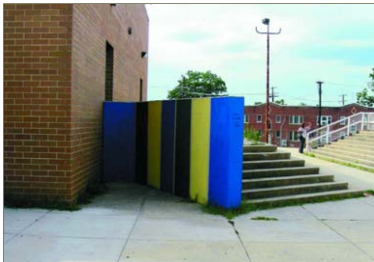
The broken sight lines on the grounds of some elementary schools, like the one here blocked by an outdoor stage, present safety issues even during daylight hours.
