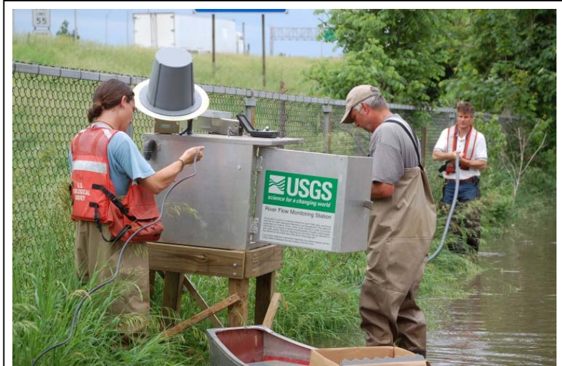
Fig. 18. USGS staff installing temporary streamgage at 13th Avenue and J Street in Cedar Rapids, Iowa, June 12, 2008. (USGS photograph by Don Becker.)
