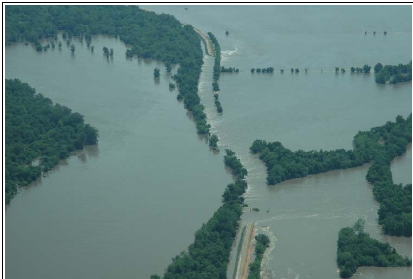
Fig. 13. Iowa River rushing through a break in the levee just upstream of Oakville, Iowa, June 15, 2008. (Used with permission. ©2008 Iowa Homeland Security and Emergency Management Division. Photograph by the Civil Air Patrol.)
