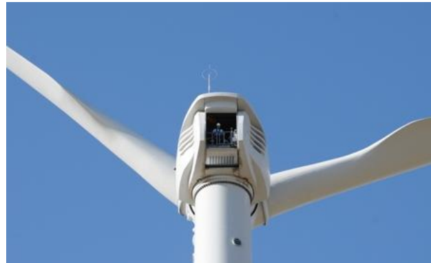
One of 97 wind towers in the Milford Wind Corridor, UT
