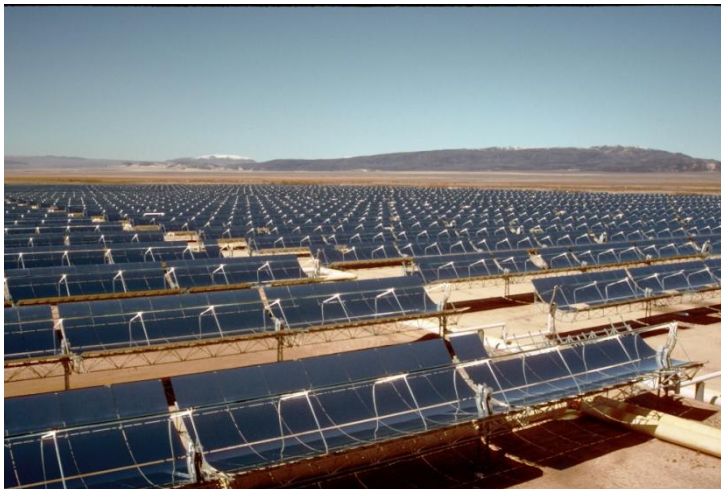
Solar array, California
