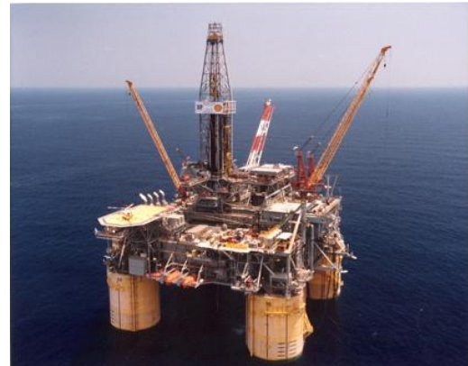
A deepwater platform operates in the Gulf of Mexico
