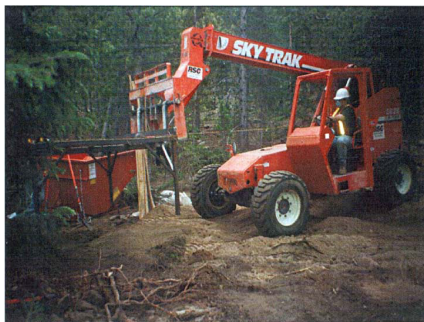
Cleanup and removal actions underway at Echo Lake Park
