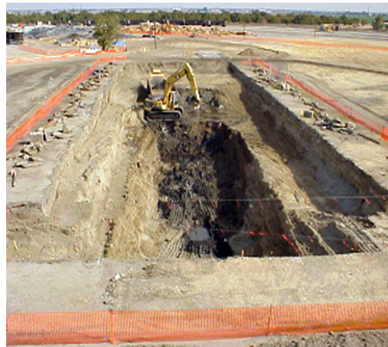
Soil contaminated with TCE undergoes remediation through soil vapor extraction
