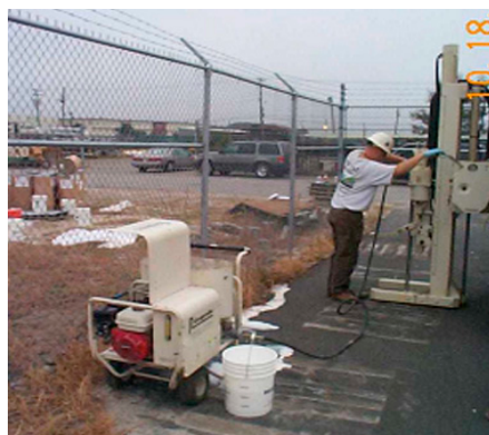
Personnel applying the ORC™ biodegradation technique at NAB Little Creek.
