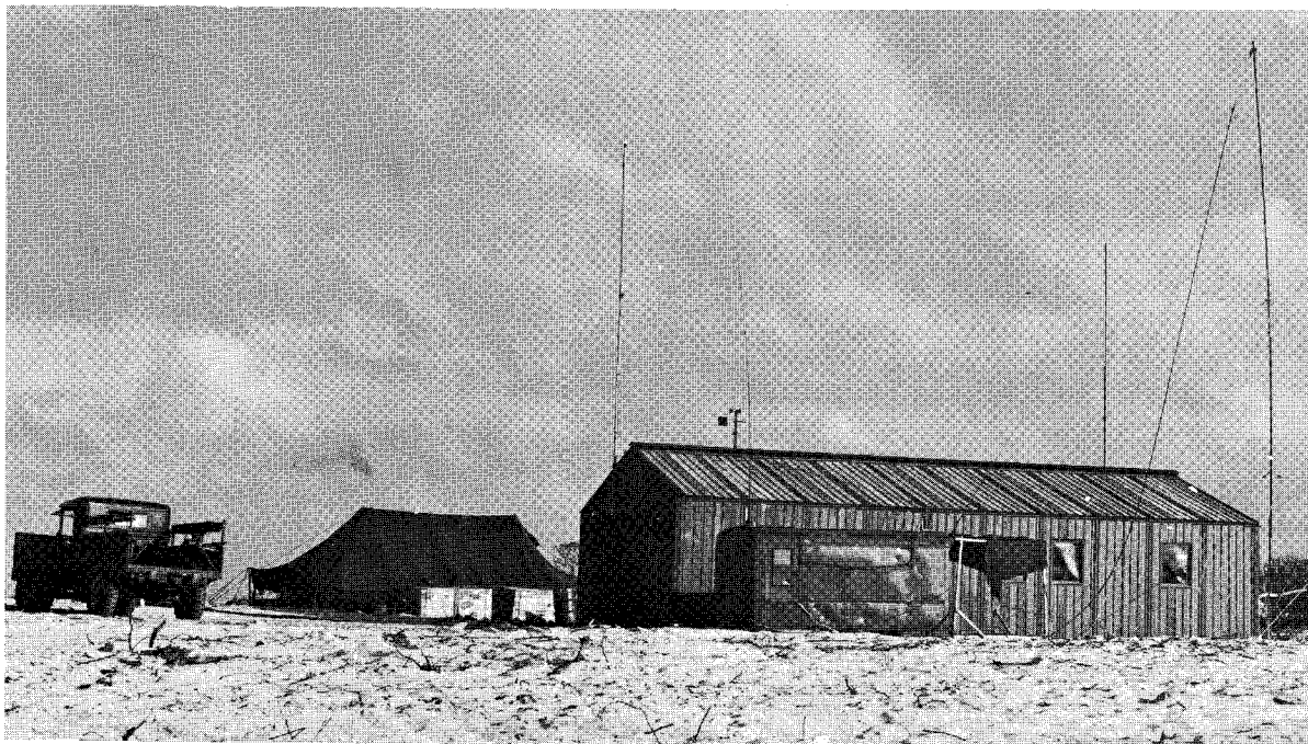
Figure 64. Photo of Rongerik installation, CASTLE.
