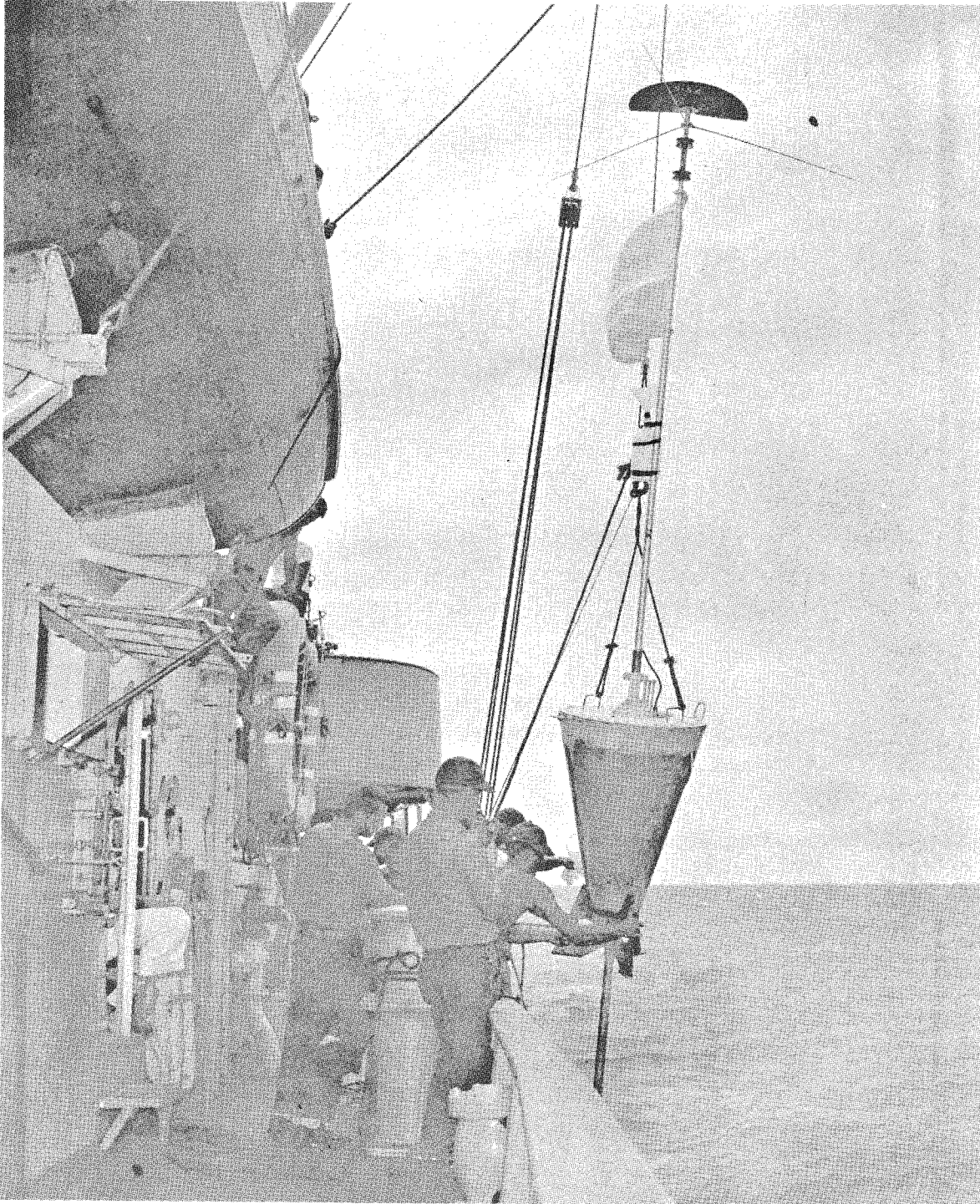
Figure 45. Placement of anchored fallout collector buoys, CASTLE.
