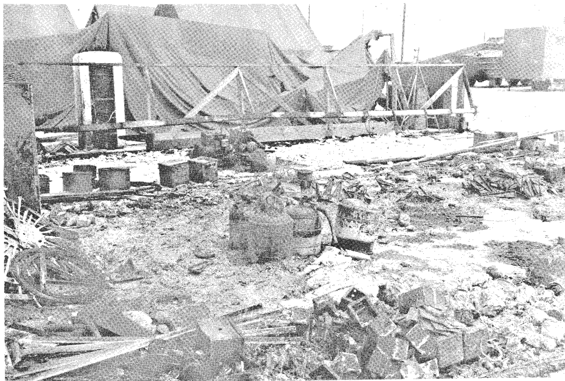
Figure 57. Fire damage at Eneman Island from CASTLE, BRAVO-induced electrical short circuit.
