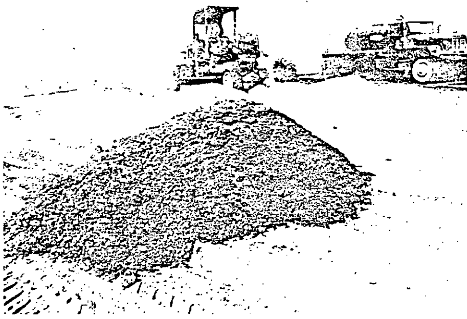
FIGURE 8-29. SPREADING SOIL WITH A GRADER.
