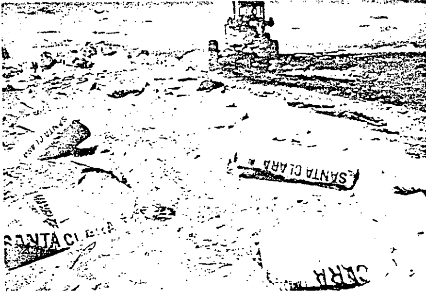
FIGURE 8-30. CEMENT BAGS PLACED FOR SOIL-CEMENT MIX.
