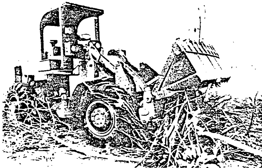
FIGURE 6-5. BRUSH REMOVAL USING FRONT LOADER.
