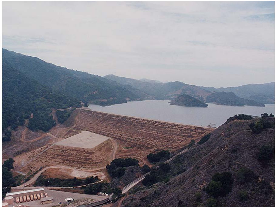
Casitas Dam and Reservoir
