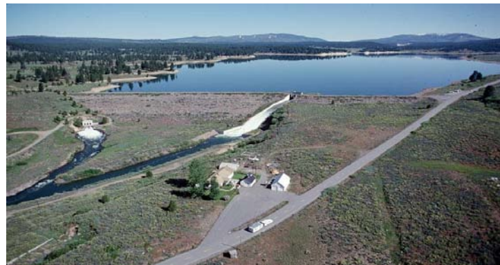
Boca Dam and Reservoir
