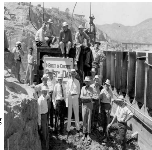
The first bucket of concrete placed to construct Shasta Dam.
