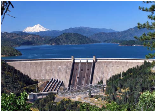
Shasta Dam and Reservoir
