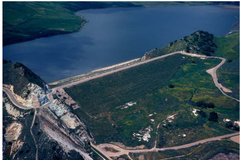
Twitchell Dam and Reservoir
