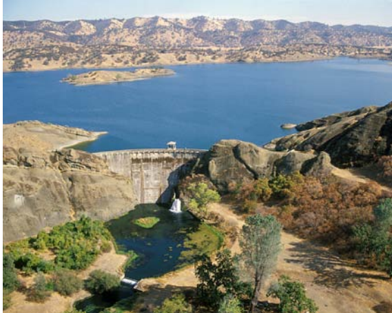
East Park Dam and Reservoir
