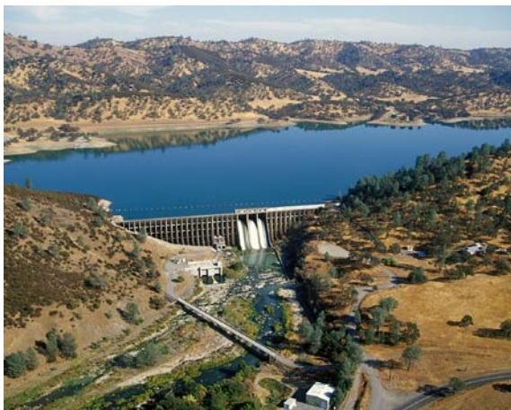
Stony Gorge Dam and Reservoir
