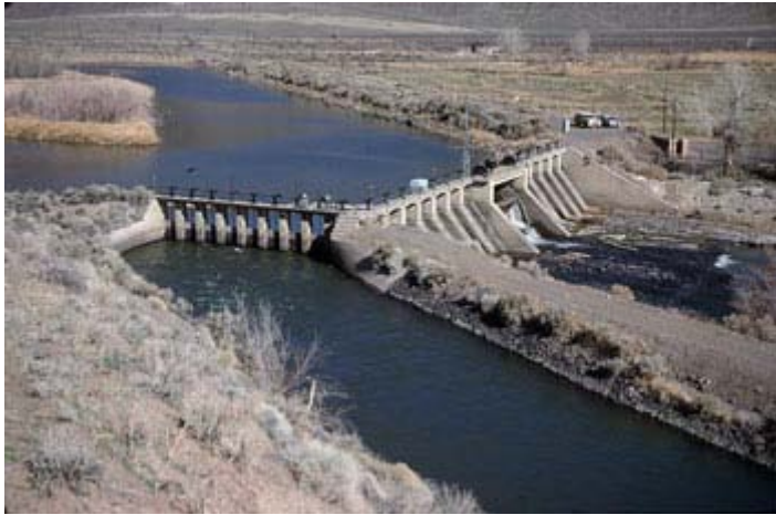
Derby Diversion Dam diverts water into Truckee Canal.
