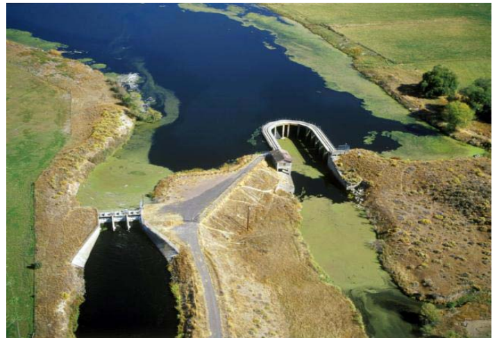
Lost River Diversion Dam is on Lost River about 4 miles below Olene, Oregon.
