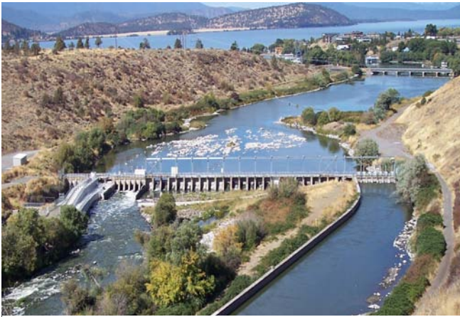
Link River Dam
