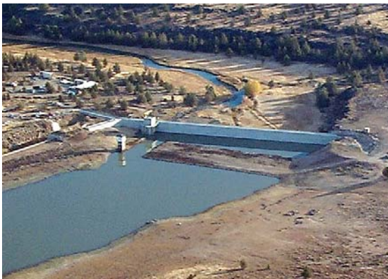
Clear Lake Dam and Reservoir
