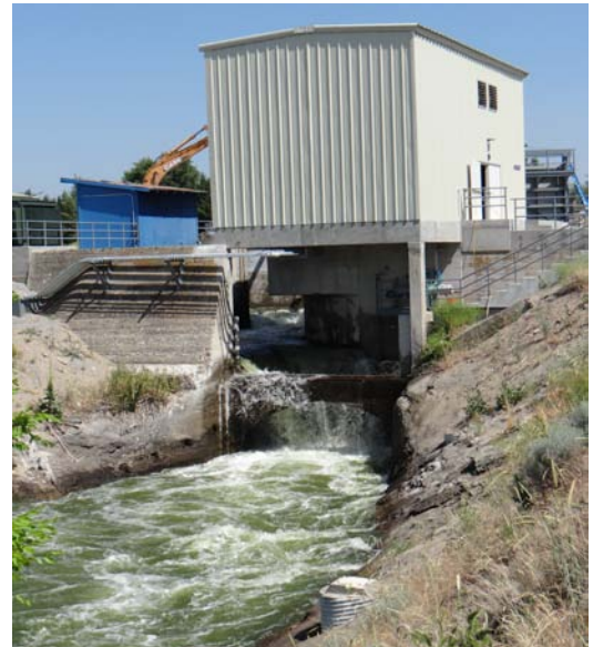
The C-Drop hydroelectric facility
