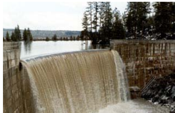
The Gerber Dam and Reservoir
