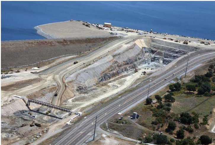
Aerial picture of the excavation of the new auxiliary spillway.
