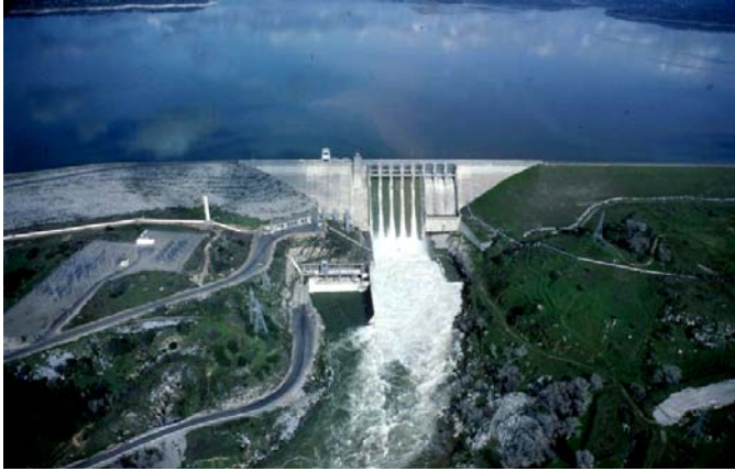
Folsom Dam and Reservoir on the American River.
