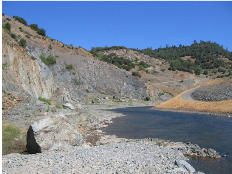
Pictured above is what the Auburn Dam site presently looks like.
