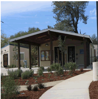
The American River Water Education Center at Folsom Dam.
