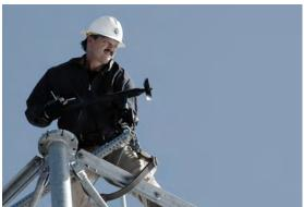
A Transmission Services employee adjusts the angle of a new anemometer, one of 14 in BPA's wind forecasting fleet. It's located atop BPA's microwave station at Sunnyside, Wash. The anemometers measure wind speed and direction, temperature, humidity and barometric pressure.
