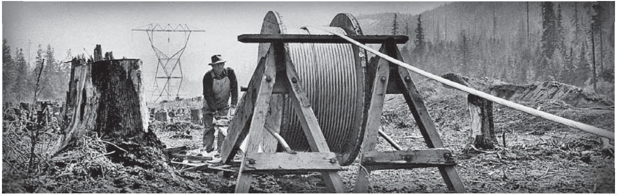
In 1942, crews strung the Grand Coulee-Covington line from eastern Washington to Puget Sound.
