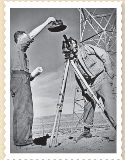
Surveying the first Bonneville-Grand Coulee line.
