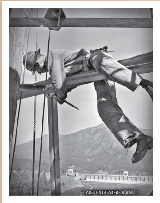
Bolting together transmission towers below Bonneville Dam ...
