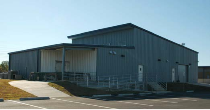
Animal Care building—housing life support area, fish kitchen, locker rooms, showers, staff meeting and records area (front view).
