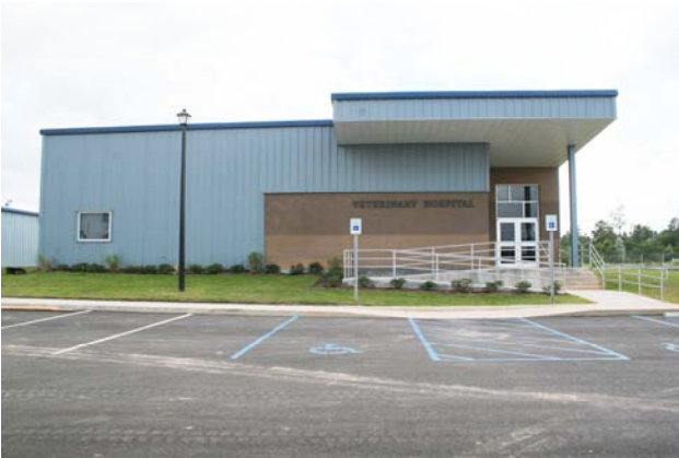
Front view (north side) of Veterinary Hospital.
