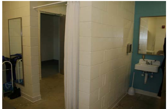
Interior view of women's locker room.
