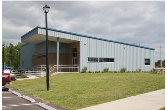
Exterior of Veterinary Hospital, north and west sides of the building.
