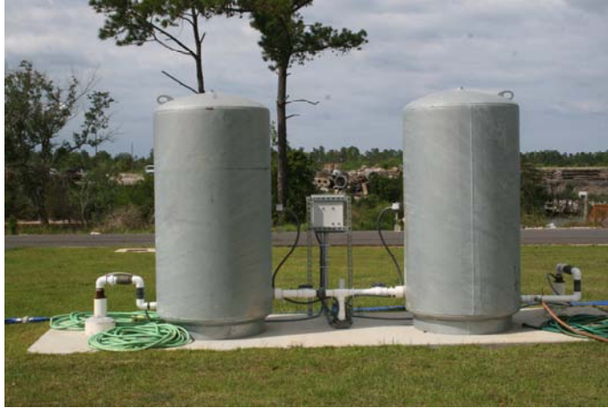
Two wells constructed for water conservation.
