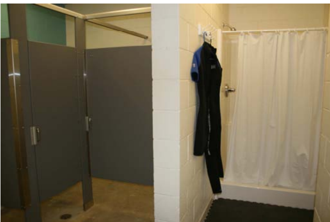
Shower and toilet facilities.
