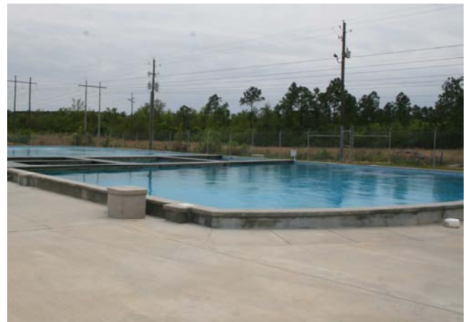
Main, large, rectangular, marine mammal rehab pool with holding and medical pens in middle. Pool capacity is 650,000 gallons and dimensions are: 125'L x 60'W x 12'D. Perimeter fence can be seen in background.
