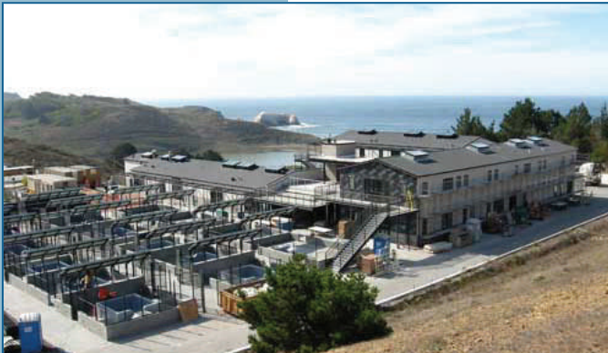
The newly rebuilt TMMC headquarters in the Marin Headlands. Photo TMMC
