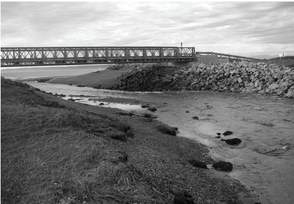
(Pictured left) The Whidbey Island Conservation District worked with NAS Whidbey Island and Skagit River Cooperative to design and build this inlet channel and beach berm.
