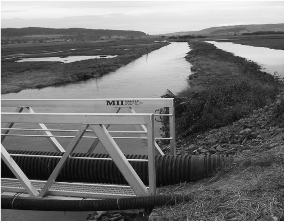
(Pictured left) 9.5 foot trestle for a sewer line crossing at the Crescen Harbor area of the Naval Air Station (NAS) Whidby Island, WA.
