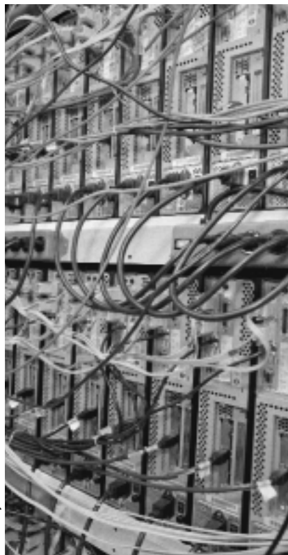
Computer specialist Don Holmgren (left) gives theorist Paul Mackenzie a tour of the new SGI machines used for simulations of quark-quark interactions. The photo on the left shows the wiring needed to let the 80 computers communicate with each other.
