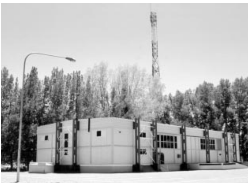
The Detector Assembly Building on the Auger Observatory Campus.
