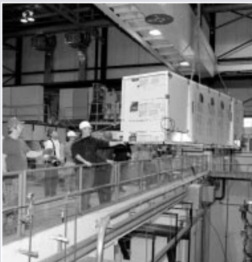
SVX aloft. CDF's crane picked up the package and swung it across the high-bay assembly hall to the waiting detector.
