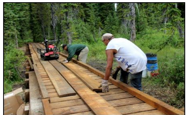
Youth Crew Works on Weitas Puncheon Boardwalk on NPNHT
