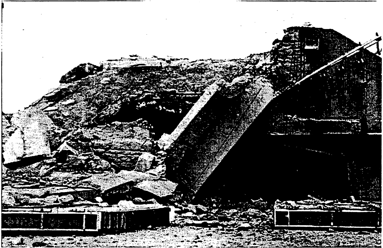
Figure 9. Close-up of Damaged Entrance to Hardened Aircraft Shelter.
